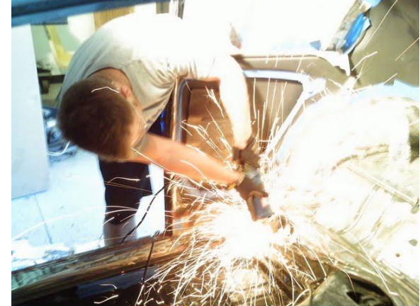
Rebuilding of VW interior for aesthetics and safety
