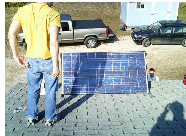
Solar panel install on “new” EcoHawks facility
